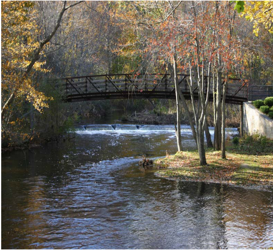
Esmond Street Park Bridge
